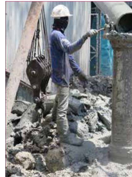
▲ Removing soft clay
