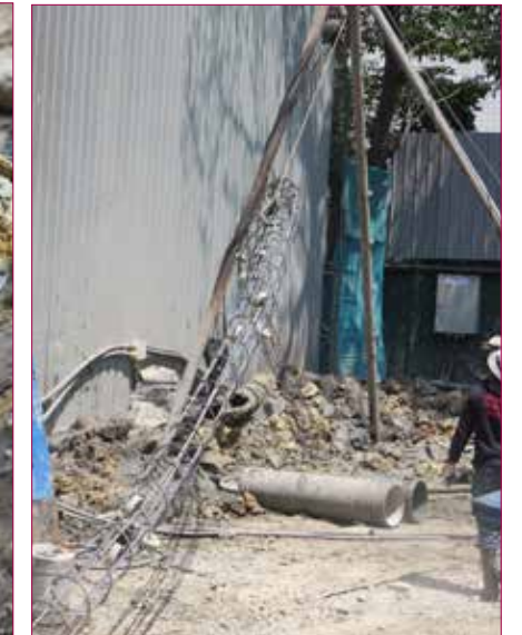
▲ Dropping cage into bore hole
