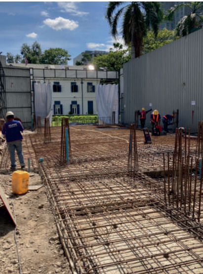
▲ Construction of ground slab
