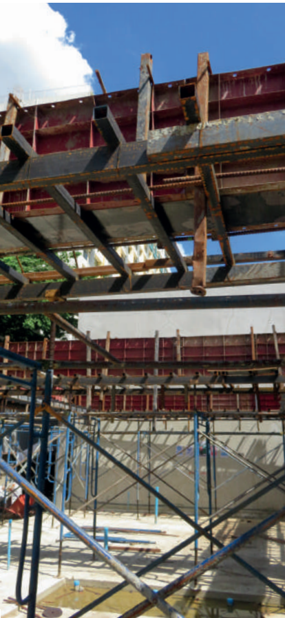
▲ 1st Floor beam framework
