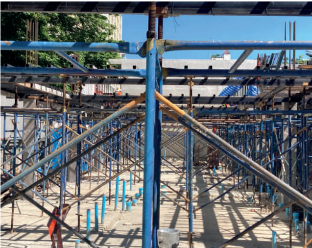
▲ Scaffolding for 1st Floor beams
