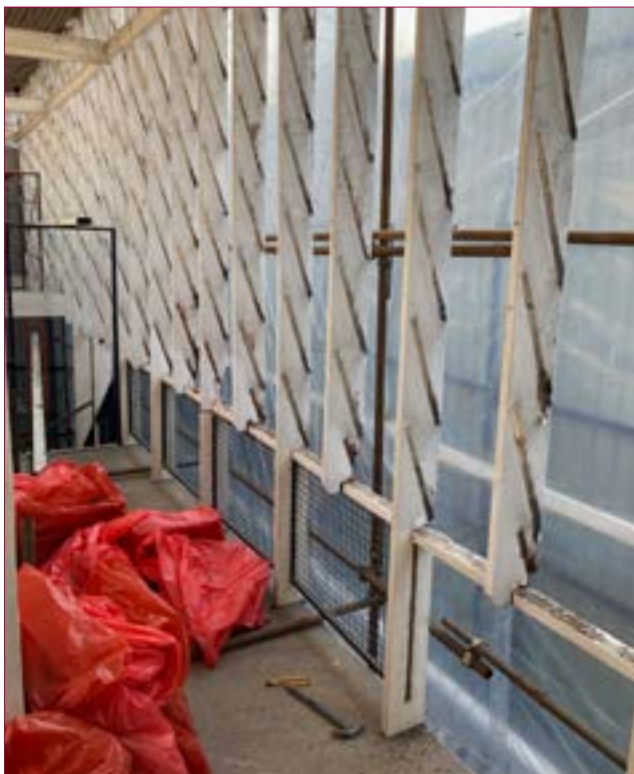
▲ Asbestos bagged for disposal
