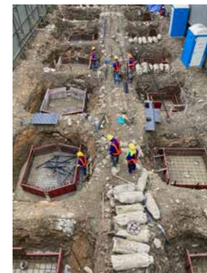
▲ Reinforcing and formwork for pile caps
