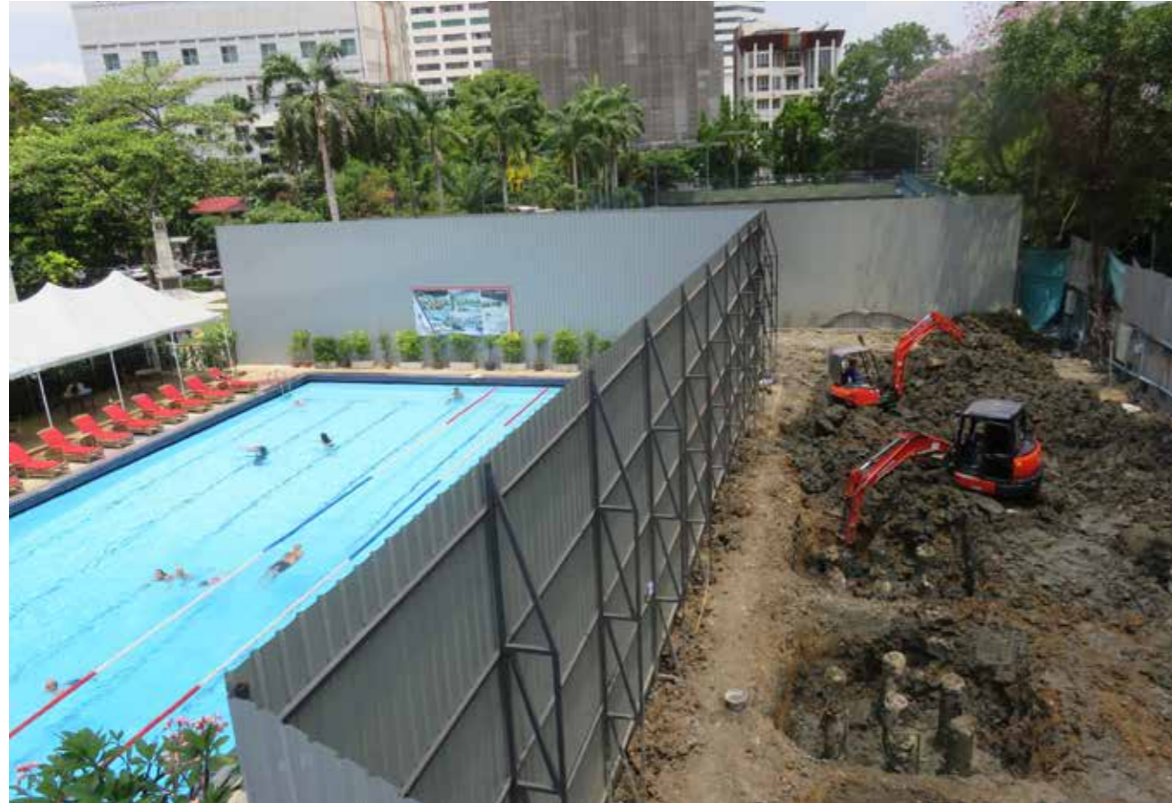
▲ Excavation of pile caps begins
