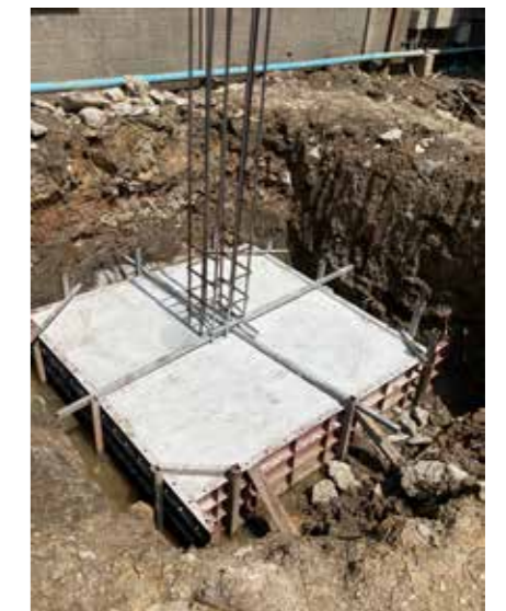
▲ Completed pile cap
