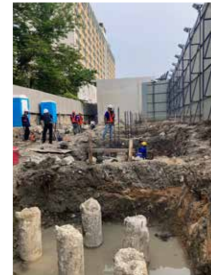
▲ Pile caps waiting to be broken out
