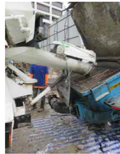
▲ Pumping concrete to pile caps
