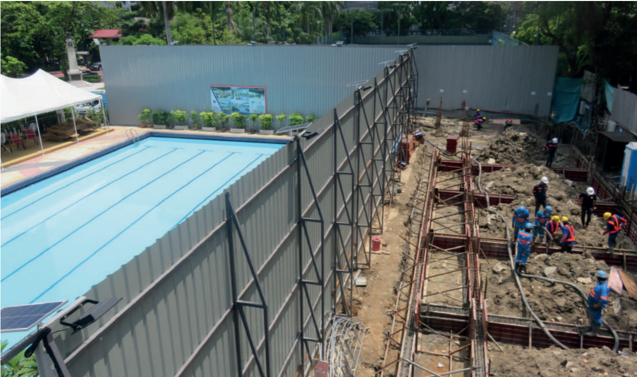
▲ Concrete being poured to Ground Beams
