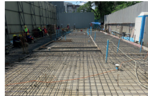
▲ Ground slabs await concrete
