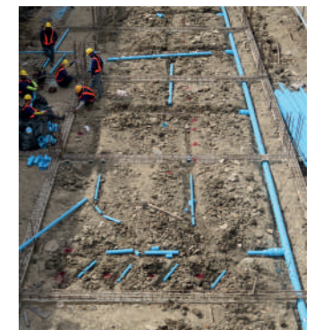
▲ Changing Room Drains
