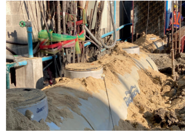
▲ Sewage Tank and Grease trap
