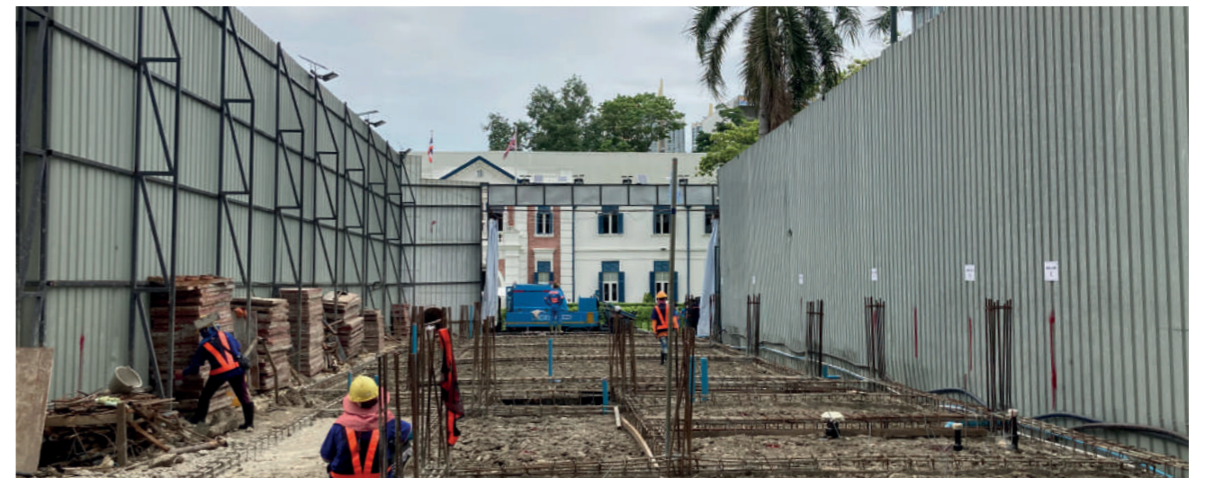
▲ Ground beams complete
