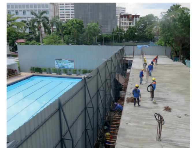
▲ 1st Floor Slab
