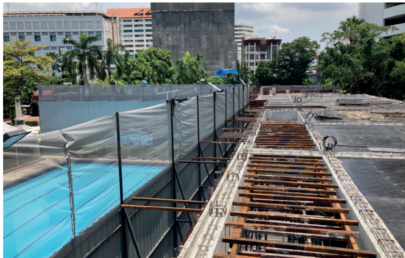
▲ Preparing for the Roof Slab
