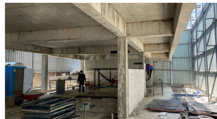
▲ First floor wall blocks
