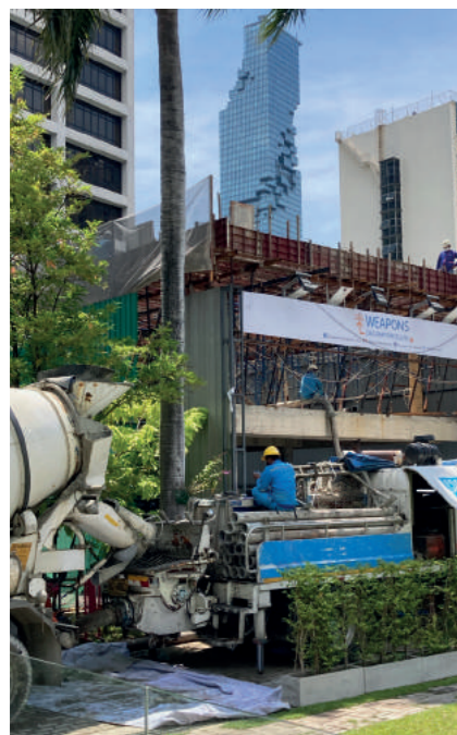
▲ Concrete delivery for roof beams
