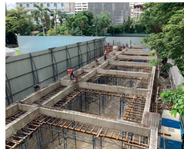
▲ First Floor Beams complete
