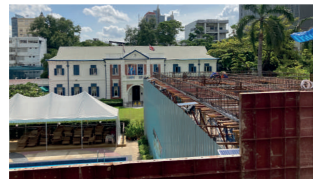
▲ Constructing Roof Beams
