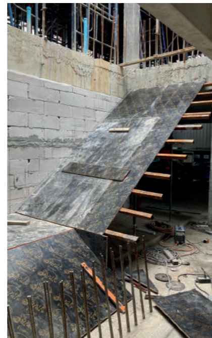
▲ Staircase to 1st Floor
