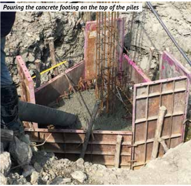
Completed concrete footing
