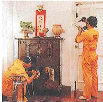
Termite control in the house
