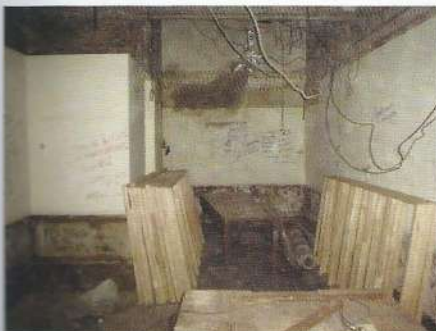
Demolition of old Churchill Bar interior – TV area
