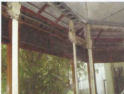
Out comes the old ceiling
