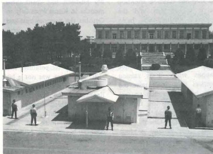
The centre hut is the negotiating room at Panmunjon on the north-south border.
