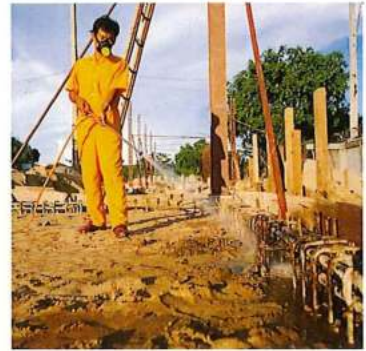
and on construction sites
