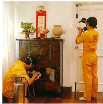
Termite control in the house
