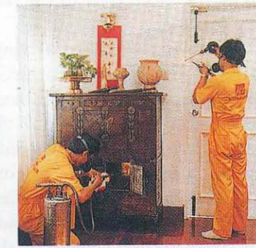
Termite control in the house
