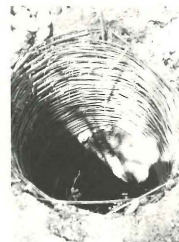
Pit with bamboo reinforced sides.
