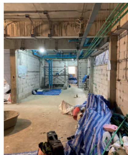
▲ Kitchen ready for plastering
