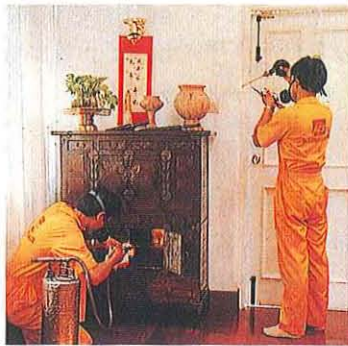
Termite control in the house
