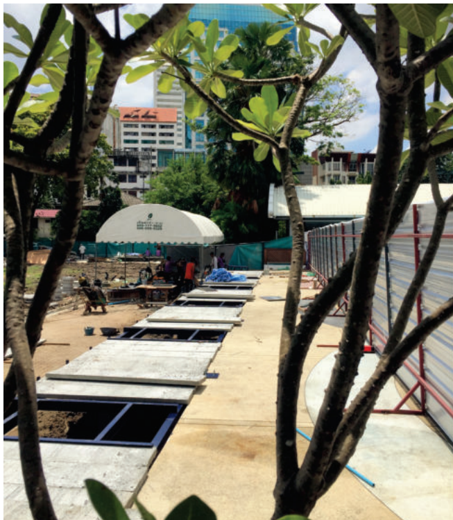
Poolside Deck takes shape
