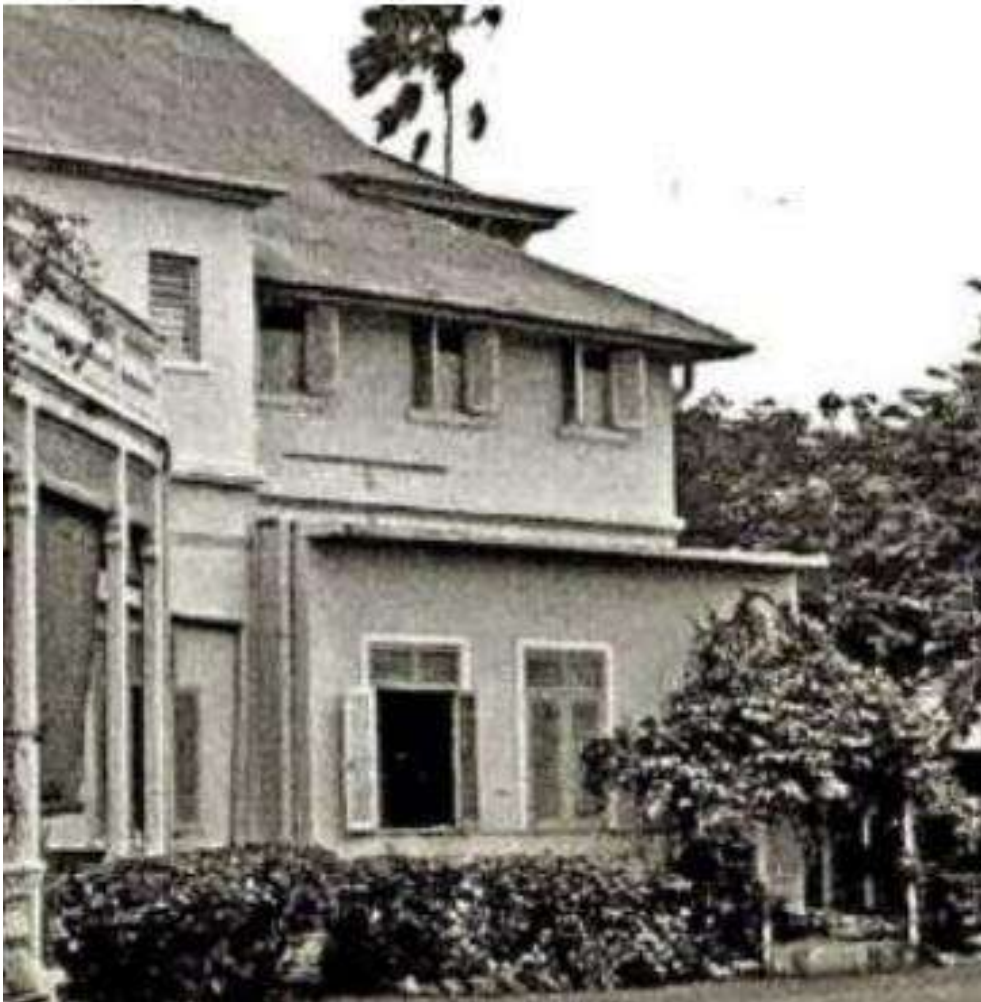
1958 image showing the rear (west) elevation with small 2m deep extension to ground floor.
