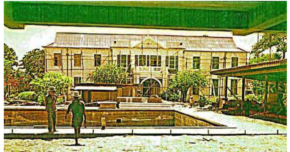
Construction of the swimming pool during the Club's major programme of expansion and modernisation in the 1960s.
