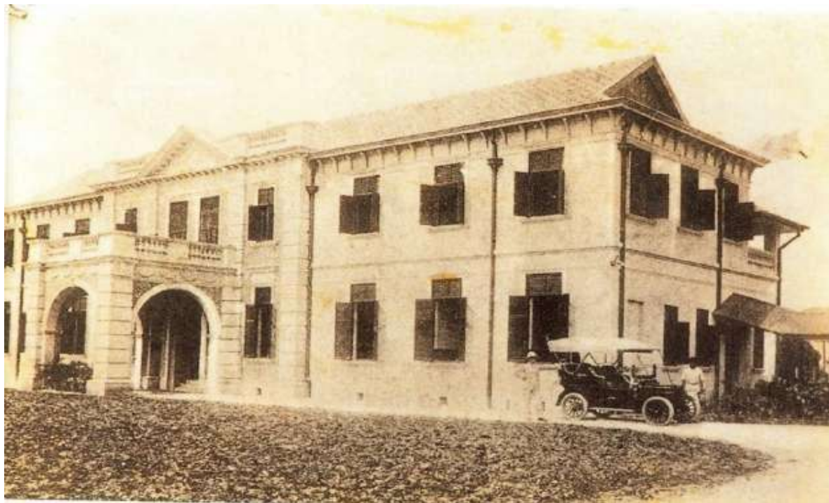
The permanent clubhouse at 189 Sunning Road, constructed in 1910 and forming the historic core of the present site.
